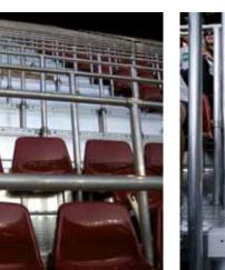
Pre-formed holes in the planks to accommodate seats and railings, greatly accelerates site assembly. The hard wearing, slip-resistant planks provide the spectators with an ideal slip-proof check.
