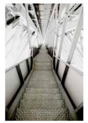
The most up to date ski jump technology for the Large Olympic ski jump at Garmisch-Partenkirchen planned and supplied by Lichtgitter. Metal profile gratings of different types ensure stability on 314 steps and 17 intermediate landings for the main staircase and on the medium and start levels and staircase near the start.
